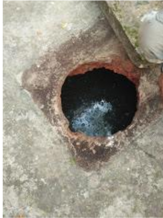
Figure 1: A Typical Soak Pit
