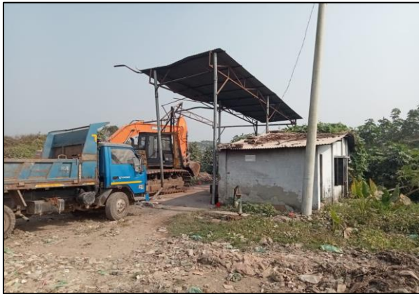
Figure 7. Site office room (H.M. Nahid, 15/12/22)
