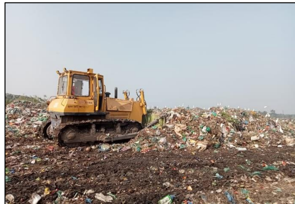
Figure 6. Leveling of dumped waste by bulldozer (H.M. Nahid, 15/12/22)
