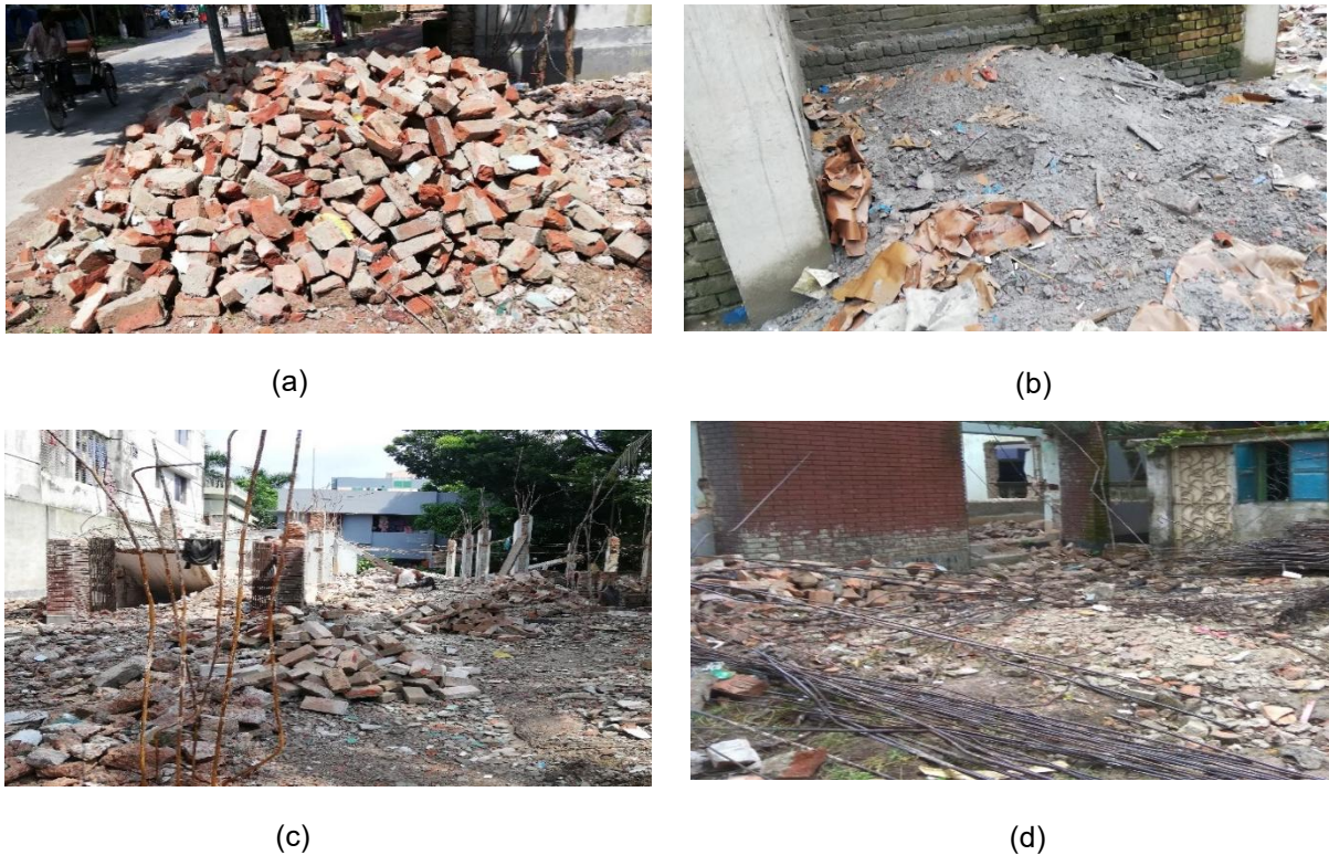
Figure 3 Waste type in C & D Process, (a) Brick Waste (b) Plaster Waste (C) Concrete Waste (d) Steel Waste
