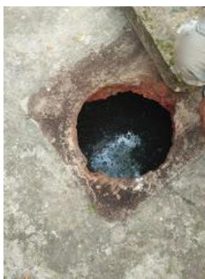
Figure 1 A Typical Soak Pit
