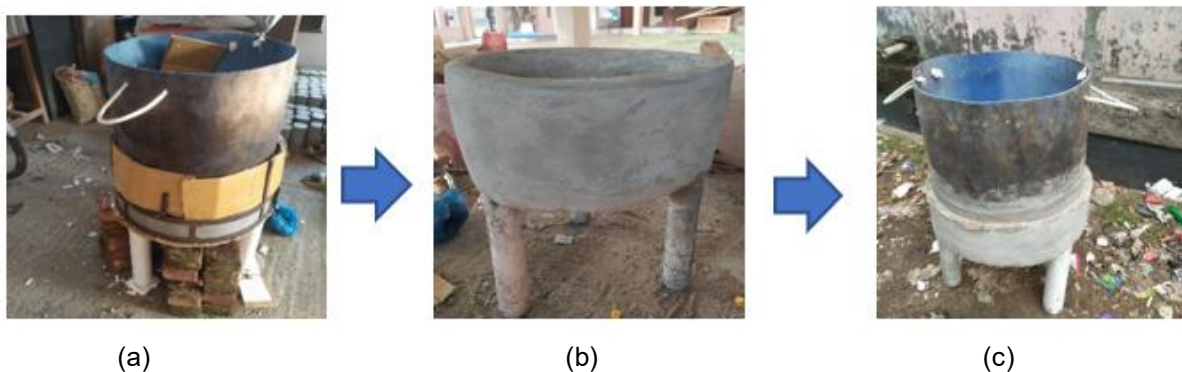
Figure 5 (a) Wastebin Holders Casting, (b) Holder without Waste-bin (After Fabrication), (c) Installation of waste bin holder in the Fulbarigate Residential Area.
